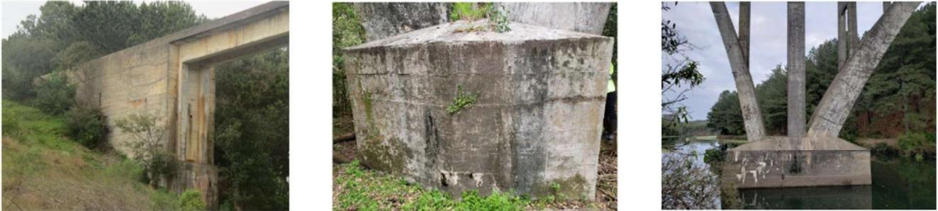
Figure 3 Substructure pathologies: concrete cracking, vegetation, concrete efflorescence
