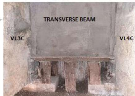
Figure 7 Emergency repair works at abutment B
