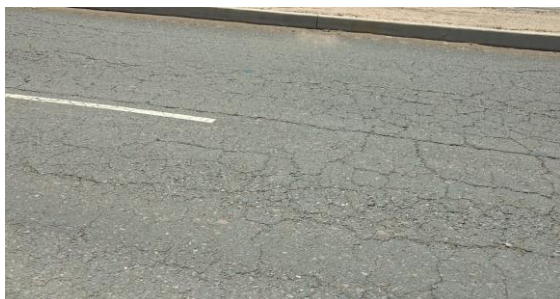
Figure 2. Alligator cracks on wearing course before the application of CGL
