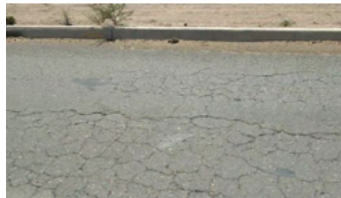
Figure 2. Alligator cracks on wearing course before the application of CGL
